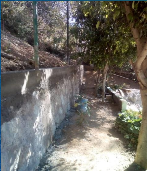
Retaining wall in school
