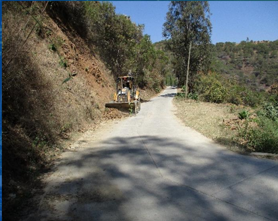
Road cleaning with backhoe
